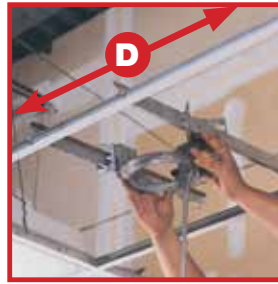
C Slide hangers with box or fixture housing attached along T Bar
